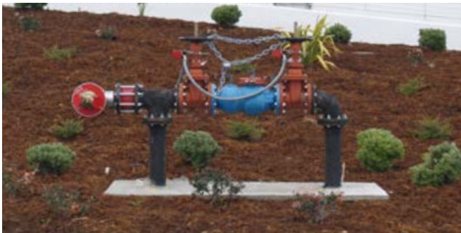
350 Double Check Valve Assembly installed to protect against backsiphonage and backpressure in low hazard applications
